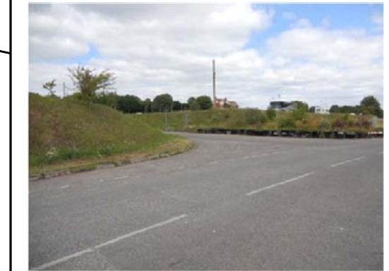
Photograph A. Junction of Bridge Road and Access Road to Turbine Site. Removal of temporary bollards necessary to facilitate ease of access.
