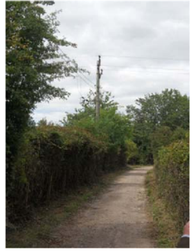
Photograph B. Access Road to Turbine Site. Removal of hedgrow to the right of photograph required. Width of track should be increased to minimum of 4.5m.
