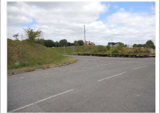
Photograph A. Junction of Bridge Road and Access Road to Turbine Site. Removal of temporary bollards necessary to facilitate ease of access.
