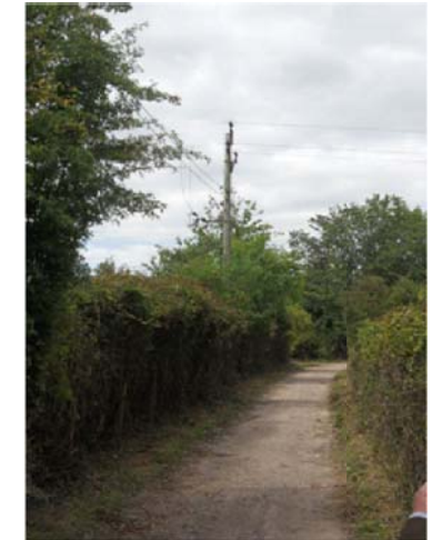
Photograph B. Access Road to Turbine Site. Removal of hedgrow to the right of photograph required. Width of track should be increased to minimum of 4.5m.
