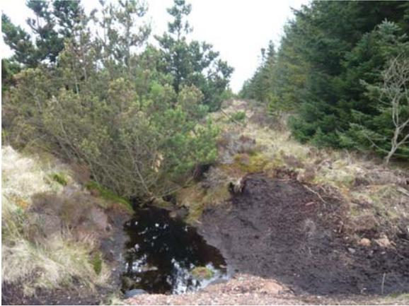
**Photo 11** Area of water draining from forestry track into drainage channel under the road and into the standing water in the mine shaft
