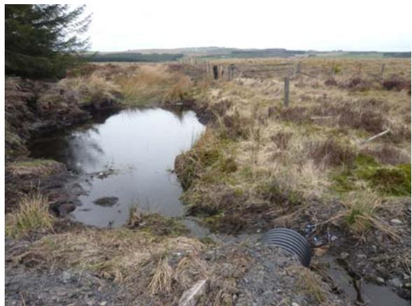
**Photo 8** Area of standing water adjacent to track, small flow through drainage channel under track. Typical of similar areas across the site
