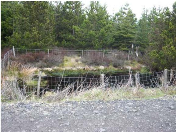
**Photo 13** Abstraction pond in case of fire, marked on OS maps as 'issues'. Water overflows in a southwesterly direction into a small drainage channel under track
